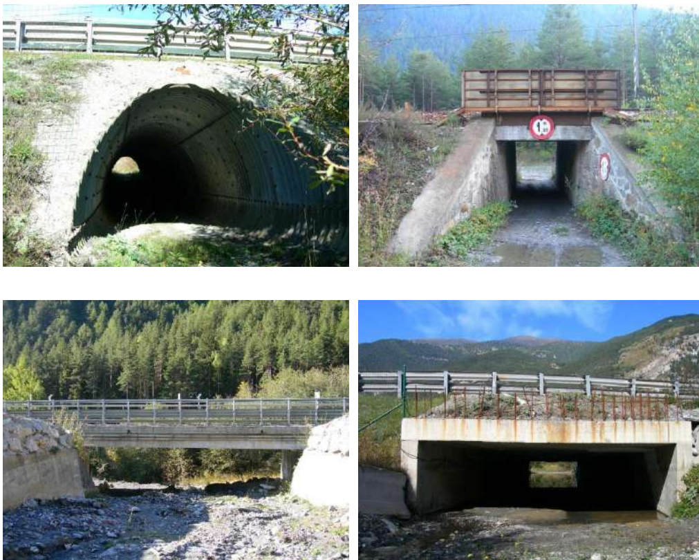
Figure15 - Road and railway line underpasses in Upper Susa Valley (Photo: Elisa Avanzinelli).
