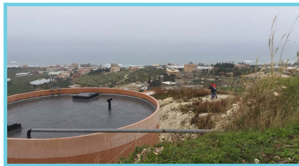
Cisterna al sud del Libano Tank in the south of Lebanon
