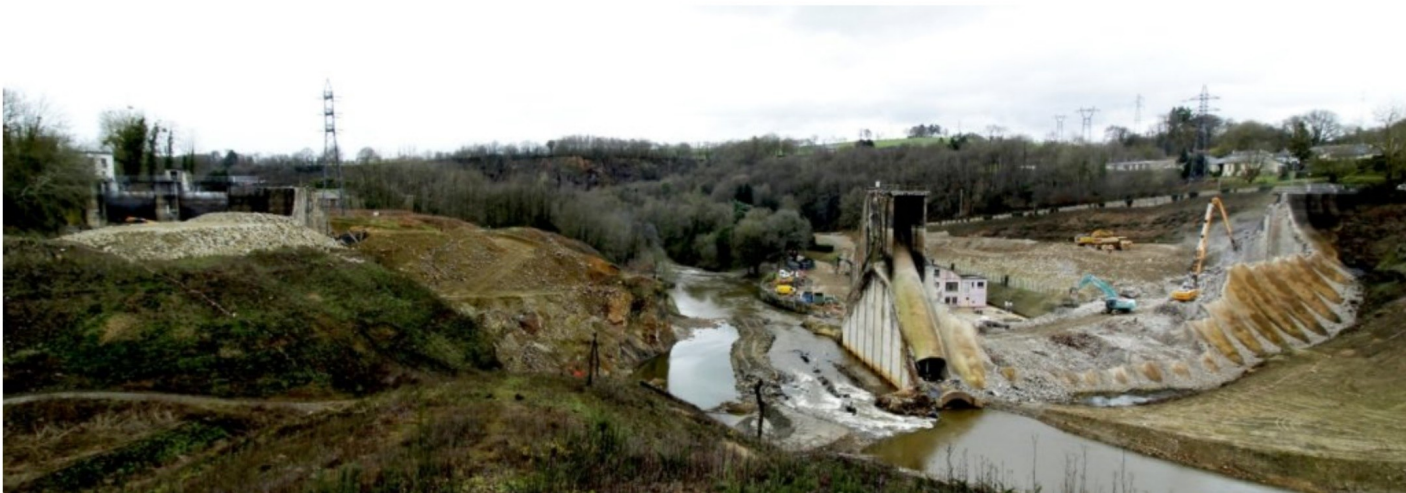
Vezins dam 13 january 2020 : 80 % of the 36 m high dam removed © DDTM50 in coop. with ERN
