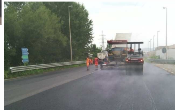
Laying of the gap-graded asphalt rubber mixture (Via Brescia – Test section 2)
