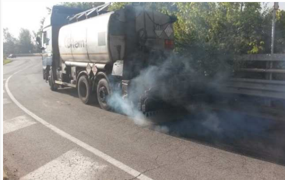
Laying of the asphalt rubber SAMI (via Brescia – Test section 1)
