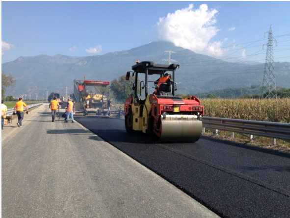
Laying of the gap-graded mixture on the SP 503 (Baio Dora)
