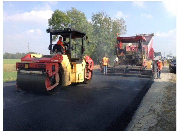
Laying of the dense-graded mixture on the SP 53 (Caluso)
