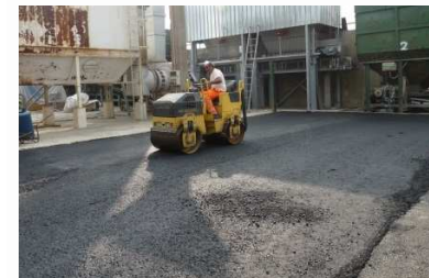
Laying and compaction of mixtures
