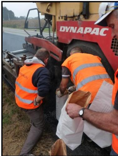
**Figure 11** – Sampling of the *dense-graded* mixture on the SP 53
