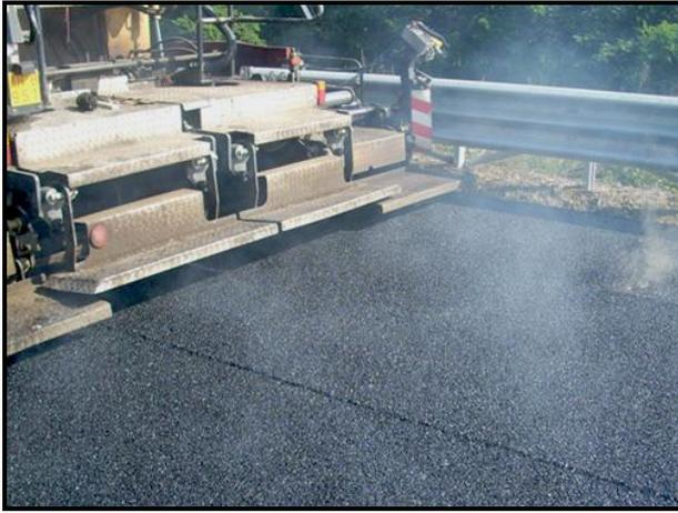
**Figure 7** – Laying of the *gap-graded* mixture on the SP 503
