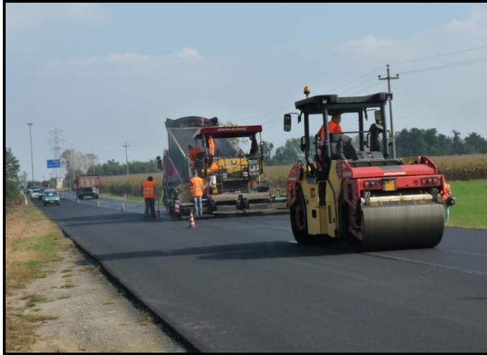
**Figure 10** – Laying of the *dense-graded* mixture on the SP 53
