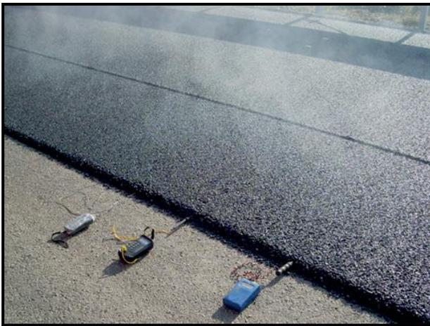
**Figure 8** – Control of compaction temperature of the *gap-graded* mixture on the SP 503
