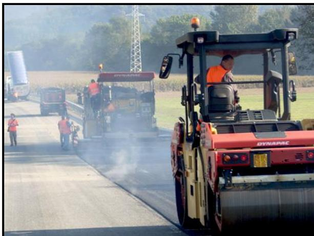
**Figure 6** – Laying of the *gap-graded* mixture on the SP 503
